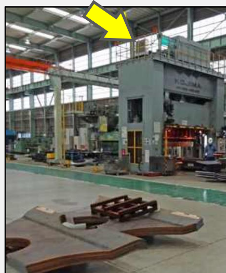
Installed in 1000t press
